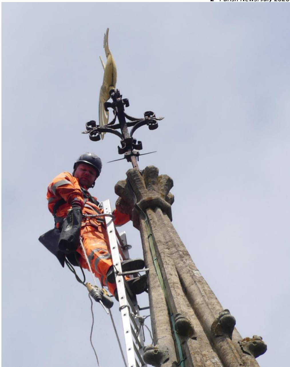
Repairing the lightning conductor on St Mary's steeple—May 2026. Picture—John Mumford
